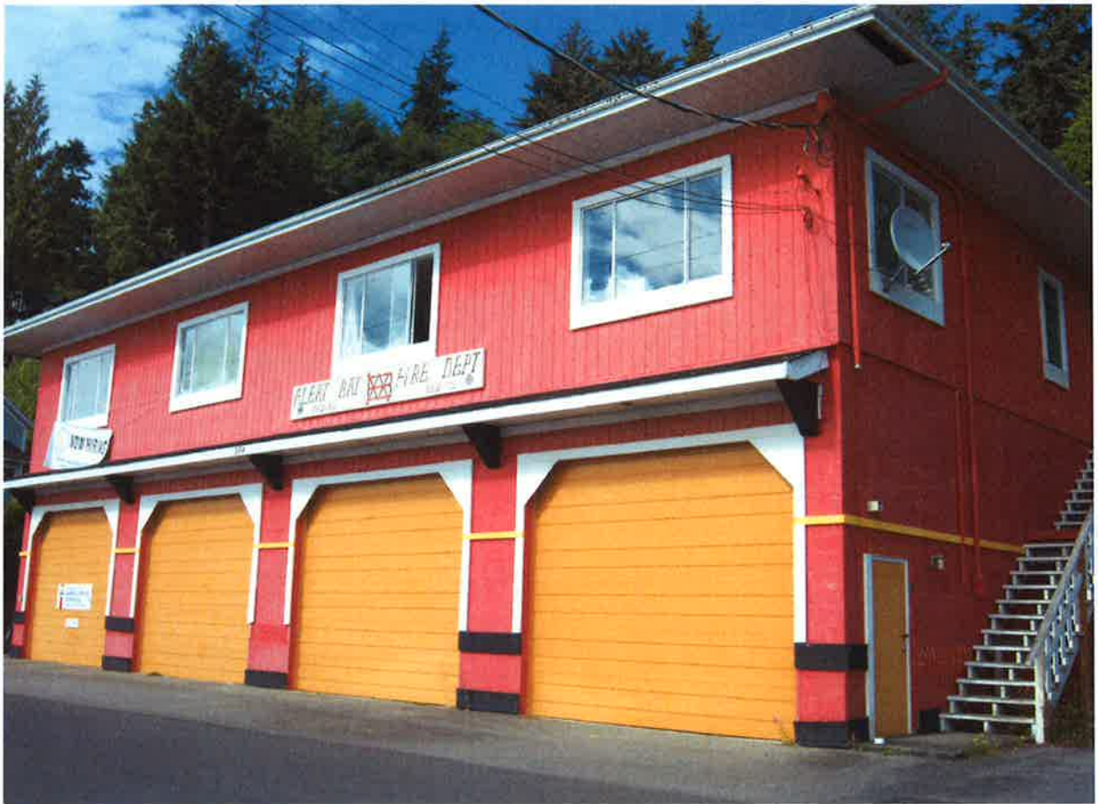
This is the Fire Hall it was completed in 1986. The old Fire Hall was the Alert Bay Visitor Centre and is now the Alert Bay Library. Kane Gordon is our local Fire Chief. There are 20 volunteer Firemen in our community.
