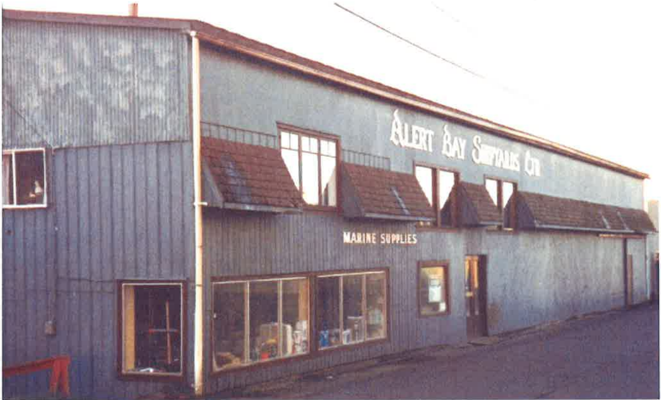
This is the Alert Bay Shipyards. The original shipyard was started in 1908 by Spencer and Huson, sons of one of Alert Bay's first settlers. Small structures have been added to it through the years. (see Historical Alert Bay brochure for more details) The Building is now privately owned.
